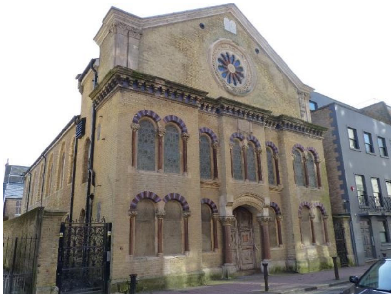
The Synagogue, Middle Street – Listed grade II*
